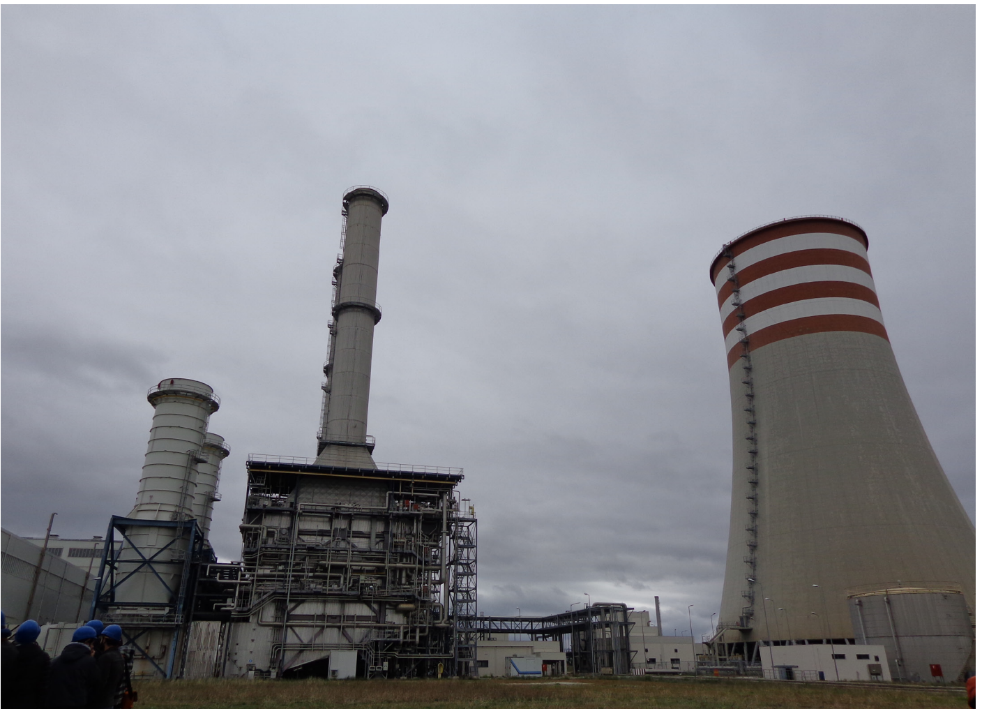
Komotini Power Plant
